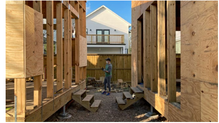
Auxiliary accessory dwelling unit (ADU) under construction in Houston’s First Ward.
