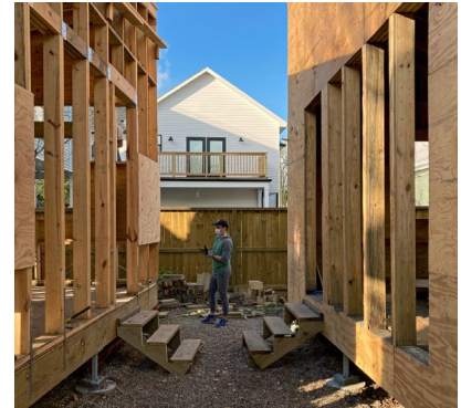
AN ACCESSORY DWELLING UNIT (ADU) UNDER CONSTRUCTION IN HOUSTON’S FIRST WARD.
